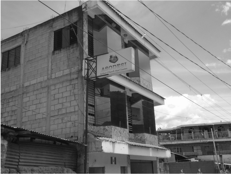
Figure 3. ASODESI offices in San Pedro, 2011. Photo by author.
