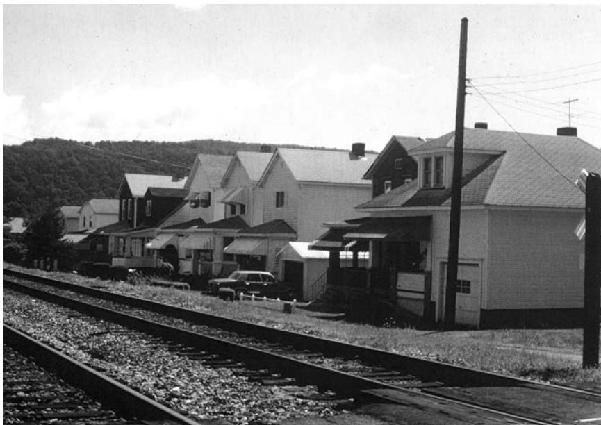
Fig. E.6. East Vandergrift. The elevated railroad bed serves as a levee. It affords some protection from the Kiskiminetas floodwaters, but not enough during extreme rainfall events. In the Saint Patrick's Day flood of 1938, most dwellings were substantially damaged or destroyed. Nevertheless, East Vandergrift, with its modest two-story houses, now represents a much safer investment for owner-occupiers than it did in the 1900s and 1910s. (Photo by Anne E. Mosher.)
