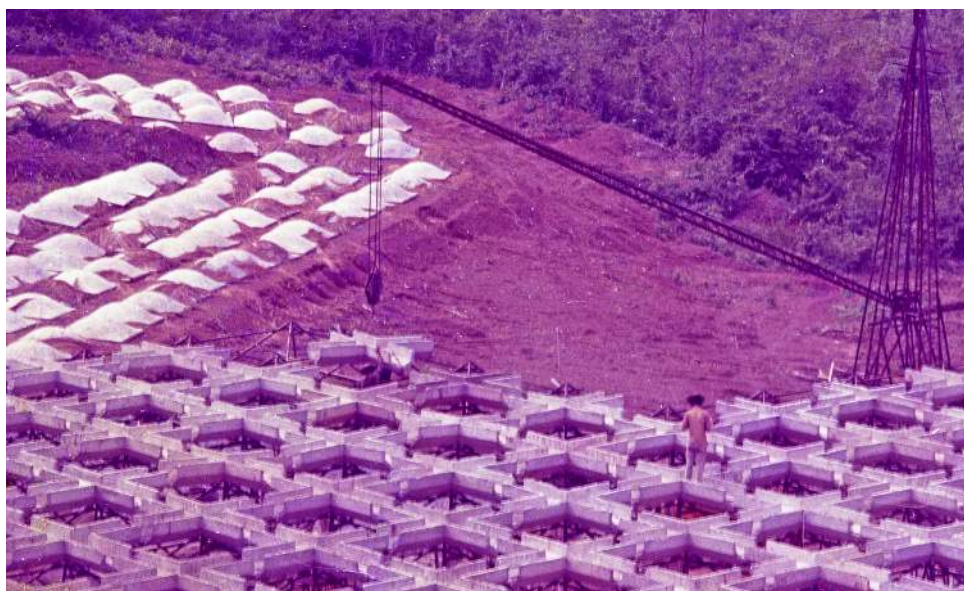
FIGURE 4: The photograph under construction illustrates particularly well how the precast elements were being made and assembled onsite. Source: Prince of Songkla University archives.
