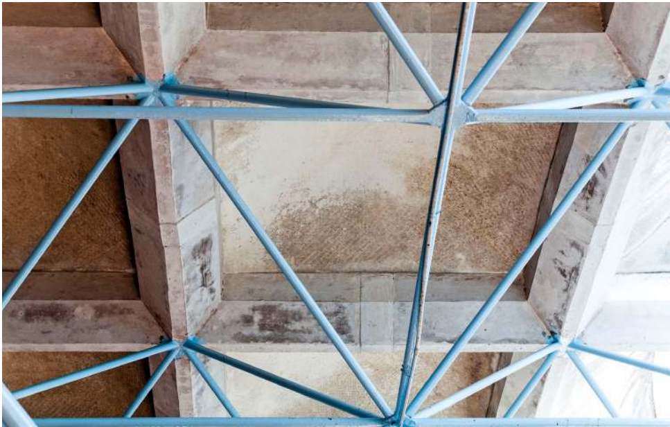
FIGURE 2: The undersides of the concrete domes, while painted, still allows the shuttering marks of lamphaen to be partially visible, giving a humanistic touch to the precast components. Source: Pinai Sirikiatikul.
