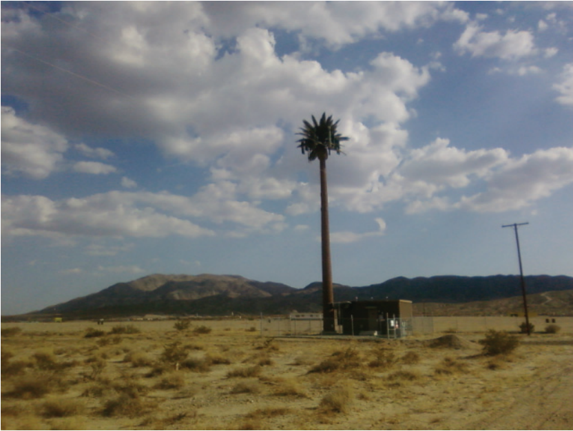
Fig. 1. Palm tree phone tower, Wonder Valley, California. Cell phone photograph taken by author, August 23, 2009.
