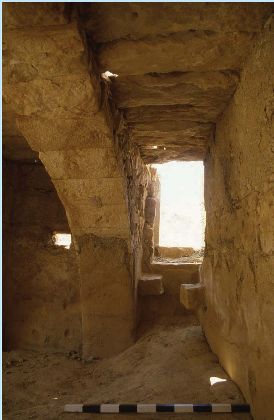
FIG. 6 The Nabataean cistern with transverse arches near Nahal Neqarot. (Courtesy of the Israel Antiquities Authority.)
