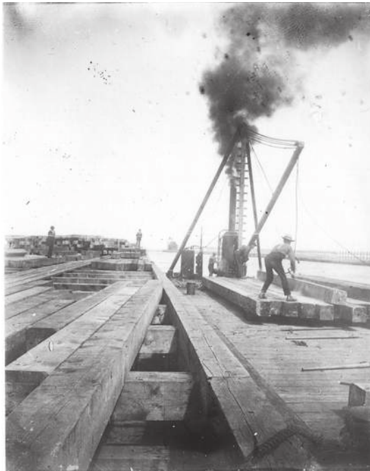
Figure 5. Late nineteenth/early twentieth-century cribwork and bulkhead construction on the channel clearing South Pier at the confluence of the St. Joseph River and Lake Michigan. Courtesy of the Heritage Museum and Cultural Center.
